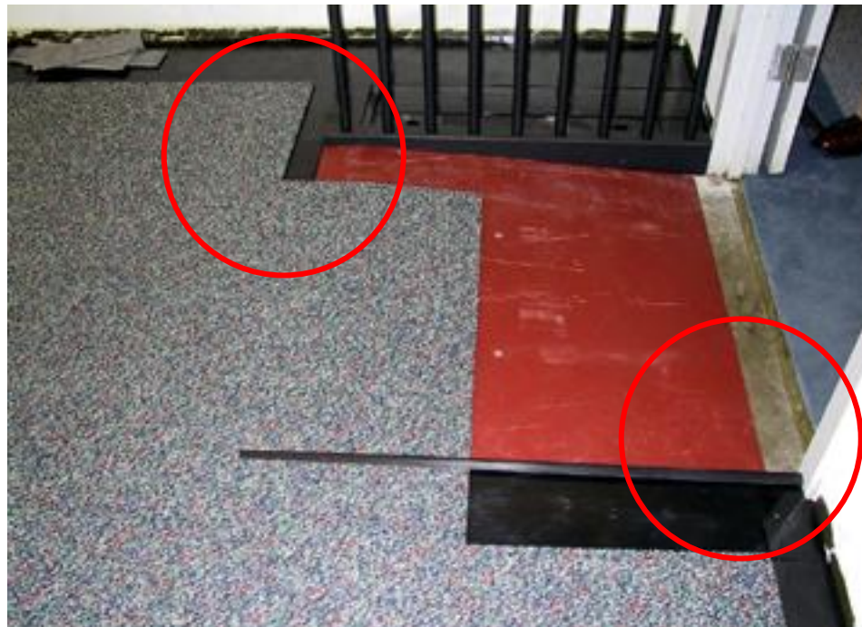
Picture 8-11 Carpet Tile seam installed beyond top and bottom of ramp
