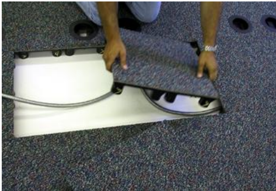
Picture 9-17 Installing completed panel into system
