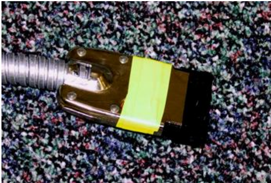
Picture 9-15 Completed Color Coding of Cable Assembly
