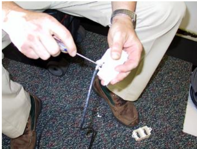
Picture 10-25 Pre-Terminated Data Cable connected to ACO Kit
