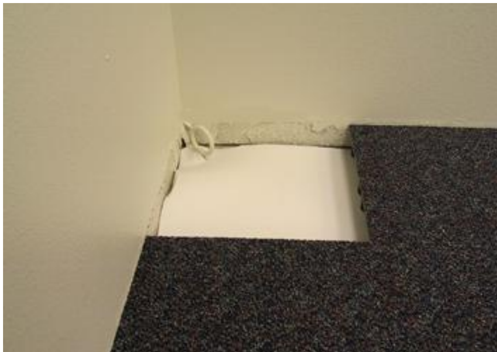
Picture 6-2 Starting the System at other than a corner
