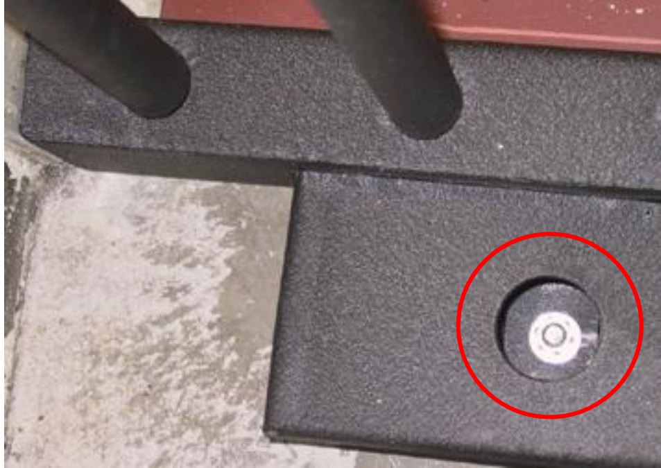
Picture 8-8 Rail anchored to floor with 2½" x 3/8" anchor bolt
