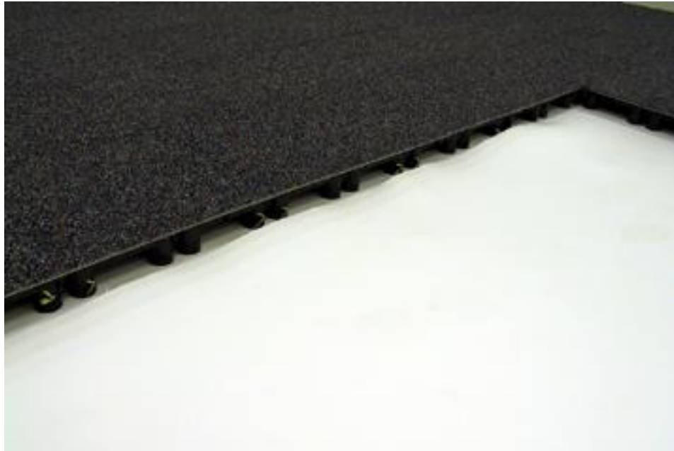
Installing Foam Underlay
