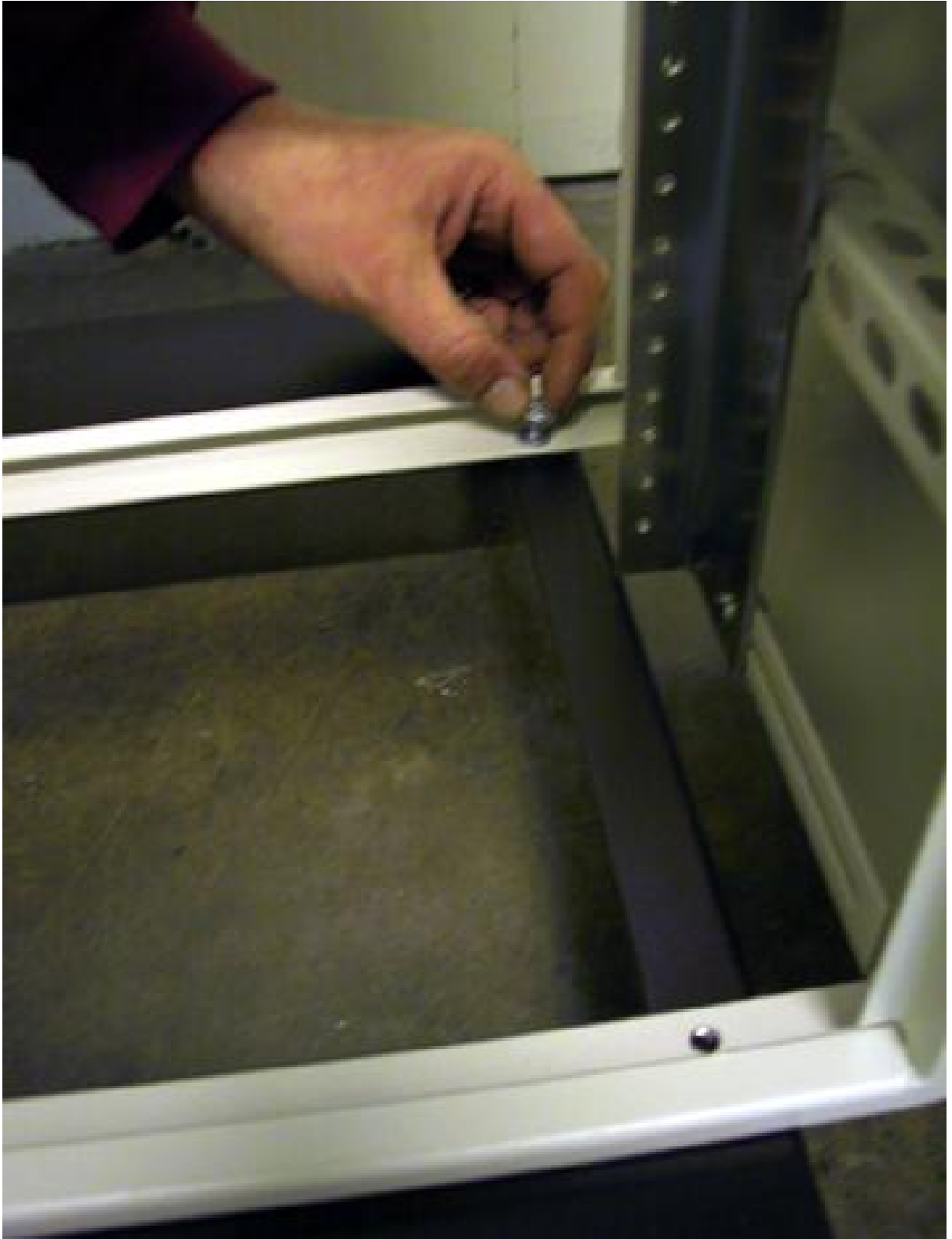
Installing LDS Cabinet to Base Unit
