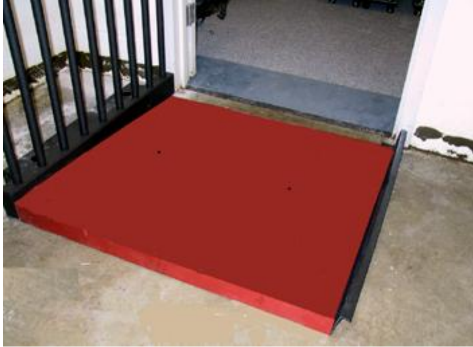
Picture 8-1 Ramp Installed with Rail and Z Trim
