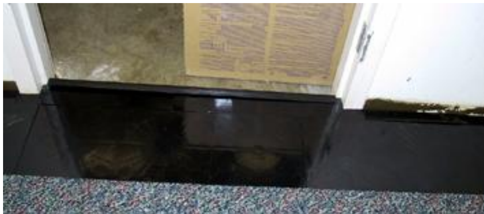
Z Trim / Perimeters in a doorway
