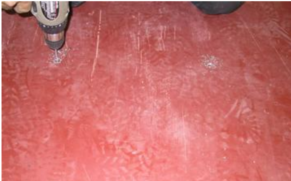
Picture 8-2 Drilling Ramp for countersunk anchors
