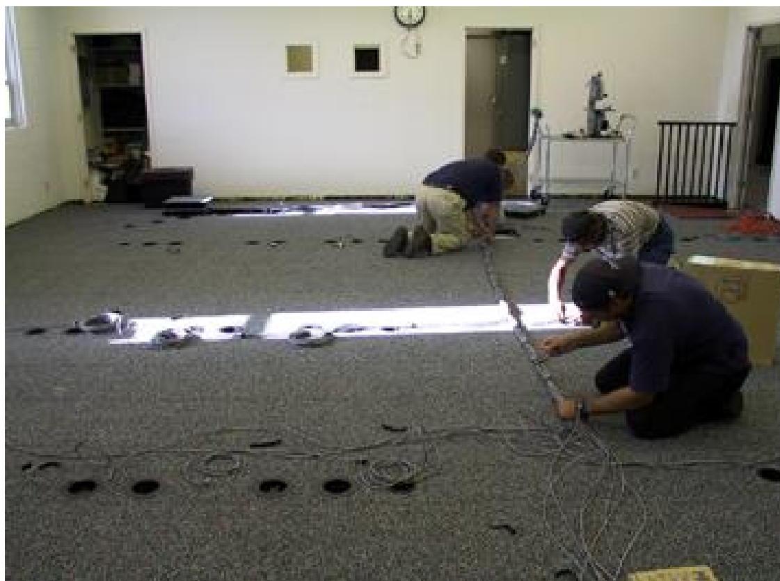
Picture 10-10 Installing Data Cables
