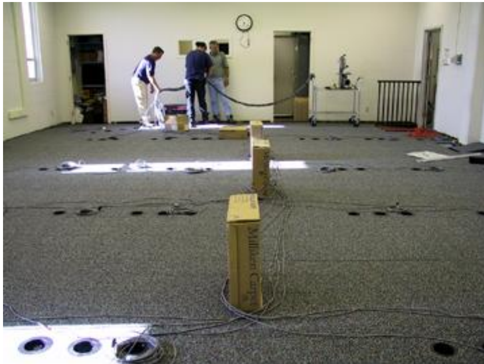
Installing Data Cables
