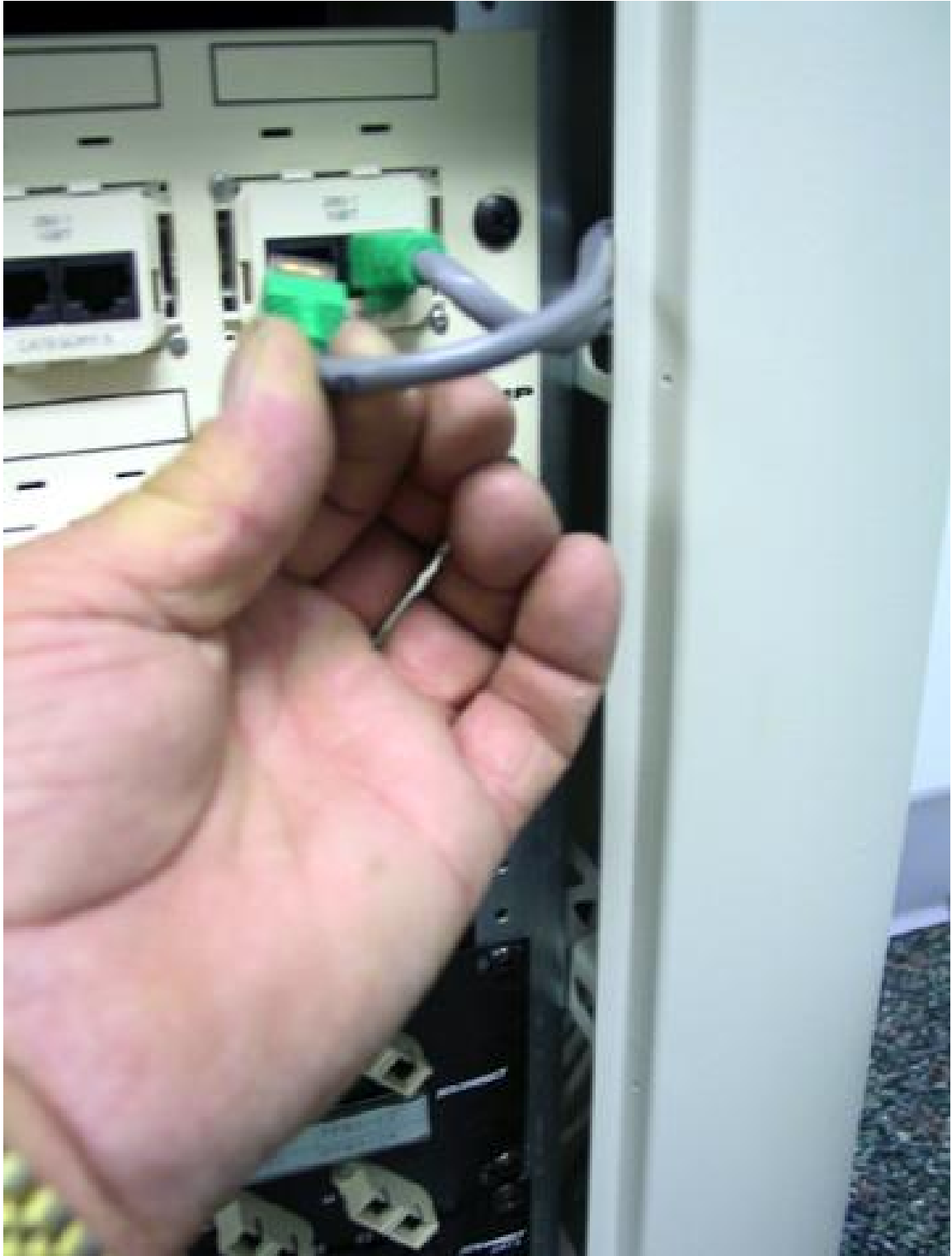
Picture 10-14 Connecting Data Cables to Patch Panel in LDS Cabinet
