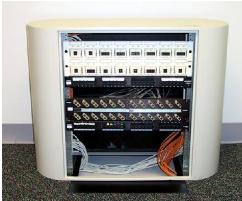
Picture 10-16 LDS Center completely installed
