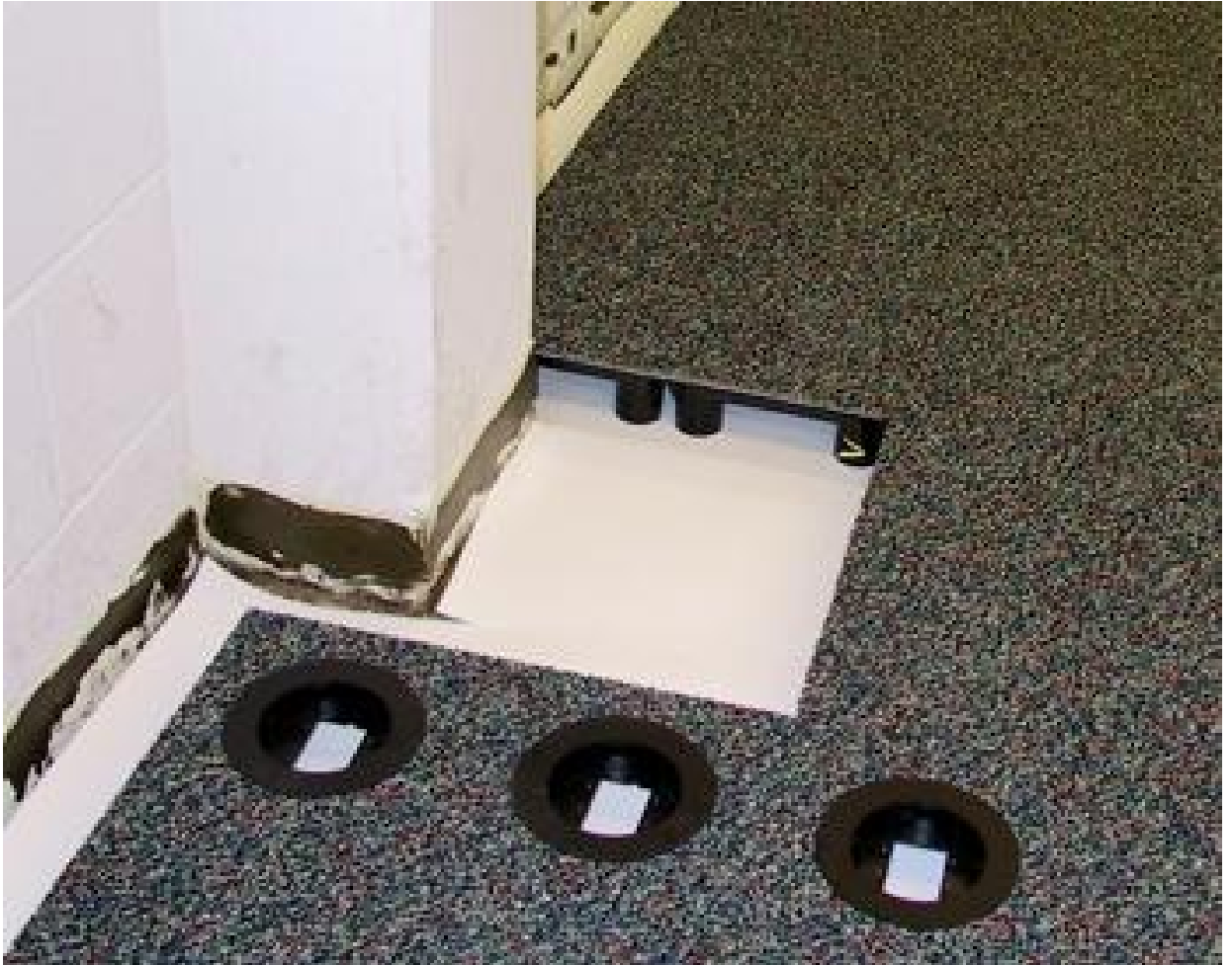
Installing the System around obstacles
