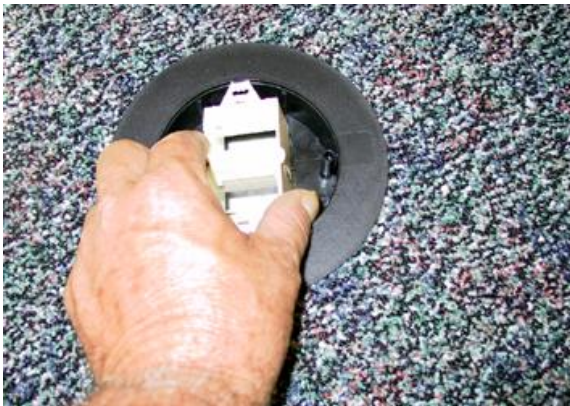
Picture 10-27 Installing ACO Kit into Powerport
