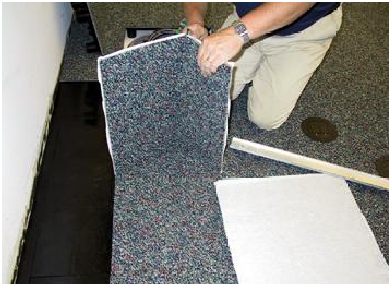
Cutting carpet tile for perimeter
