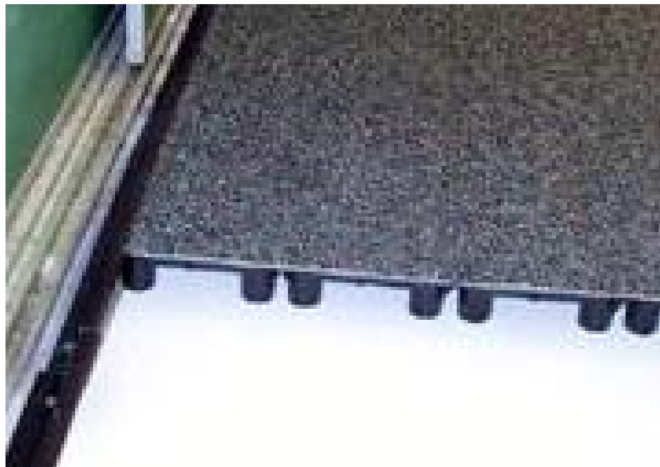
Z Trim installed at the edge of the system
