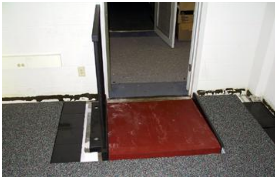
Picture 8-9 Rail, Ramp, and Z Trim mounted to floor
