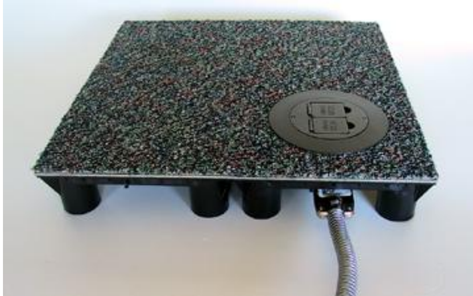
Picture 9-16 Completed Panel with Cable Assembly connected
