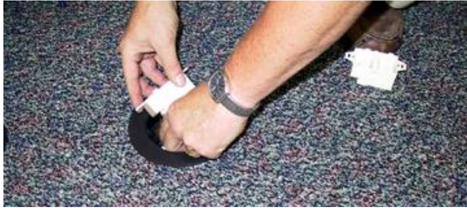
Picture 10-27 Installing ACO Kit into Powerport
