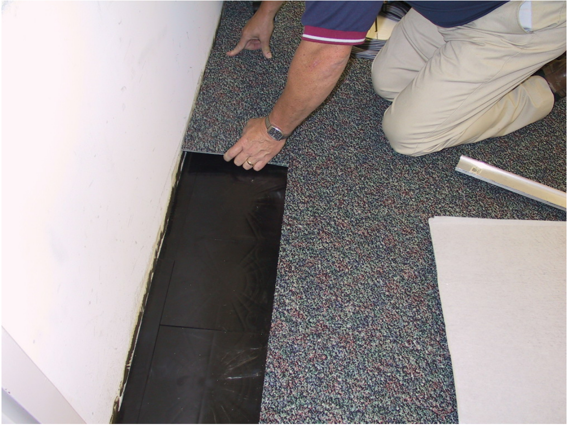
Installing carpet tile on perimeter
