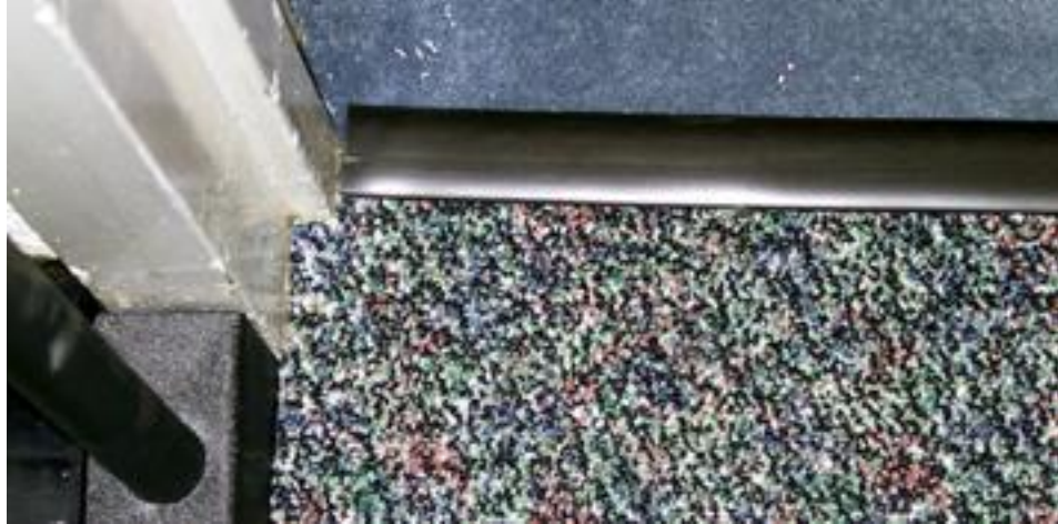
Installed Transition Molding
